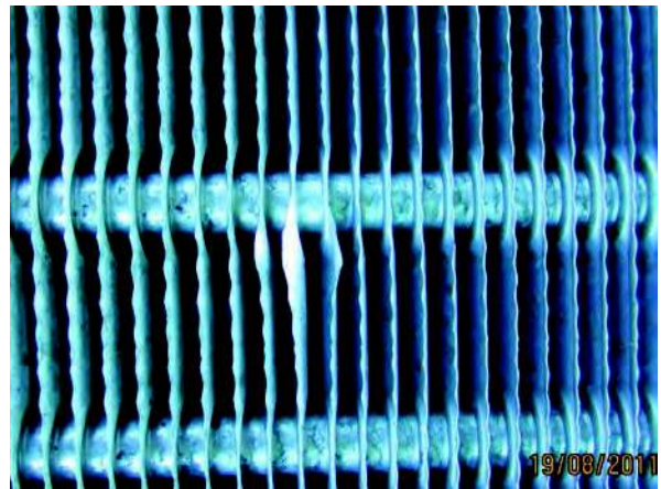
Coil after cleaning
