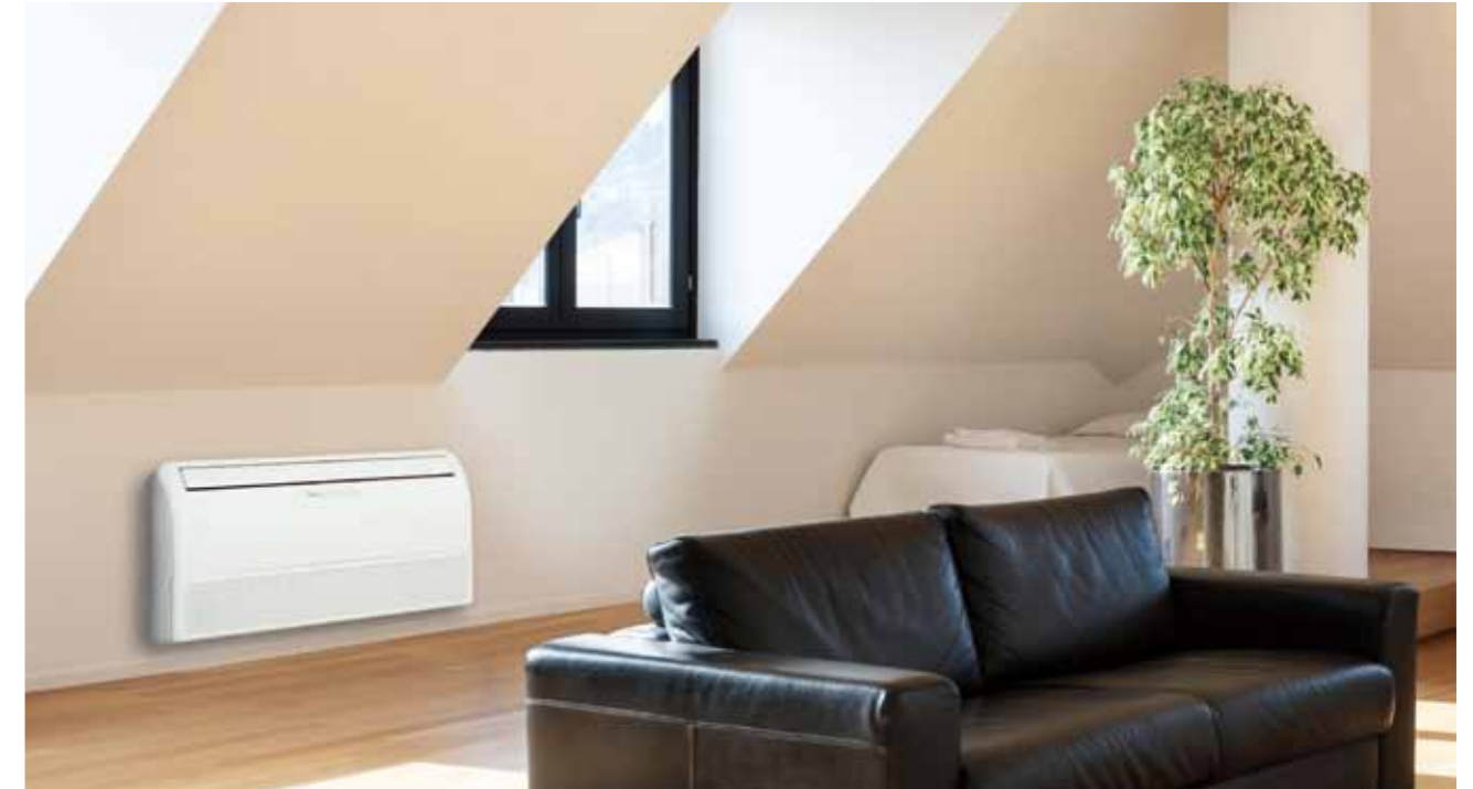
The floor-level installation
